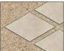
Laying on sand
