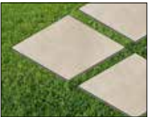
Laying on soil / grass
